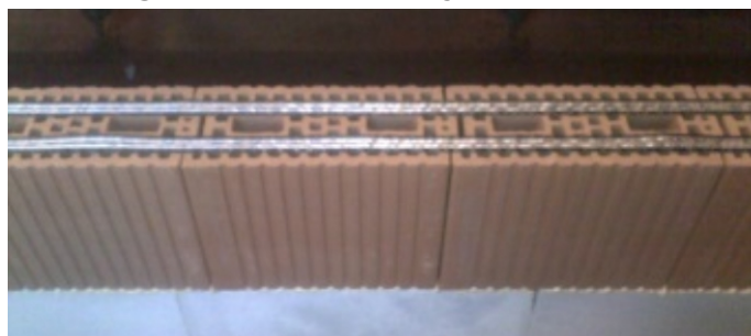
Figure 16 – Armature de joint horizontal
