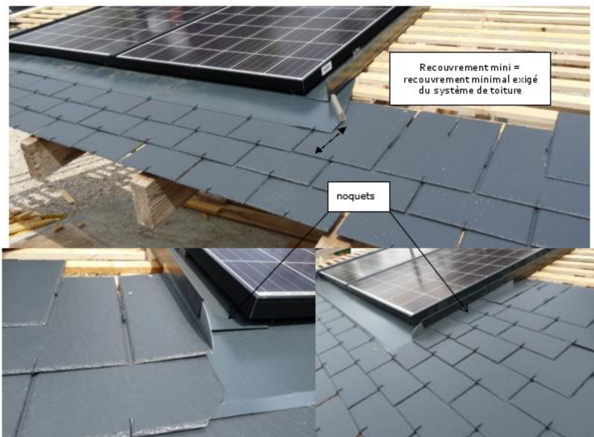
Figure 59 – Recouvrements inférieurs – kit PV3-1 TP/Ardoise
