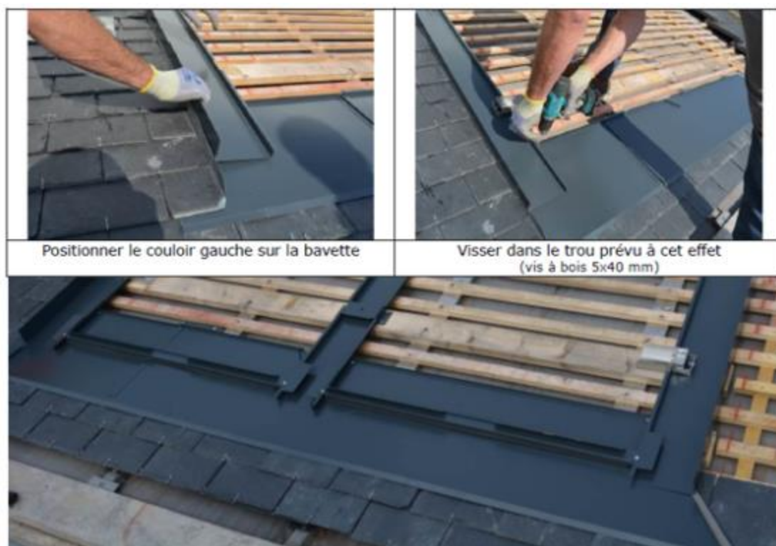
Figure 48 – Montage des couloirs – kit PV3-1 TP/Ardoise
