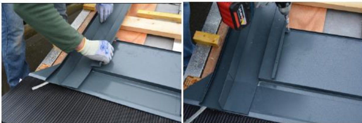
Figure 47 – Montage des couloirs – kit PV3-1 N
