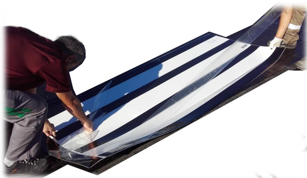
Figure 2a – On retire le film pelable des bandes Butyle
