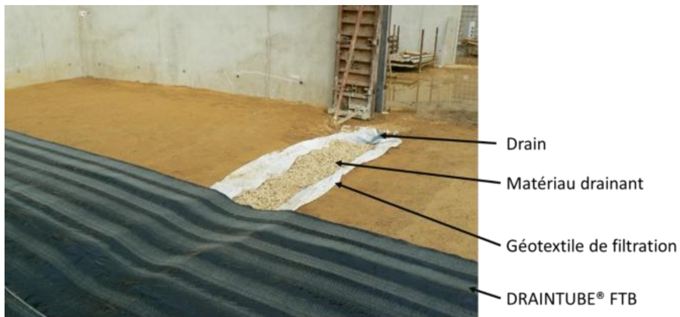
Figure 2 - Raccordement DRAINTUBE® FTB / tranchée drainante
